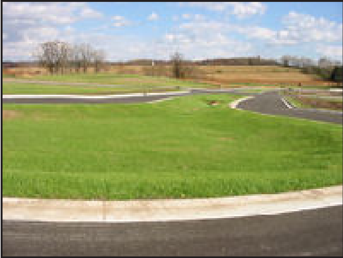
Figure 6.130: Infiltration Basin. Source: University of Wisconsin Extension
