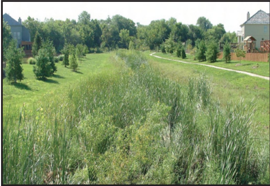
Figure 6.115: Wetland Swale. Source: Olsson Associates
