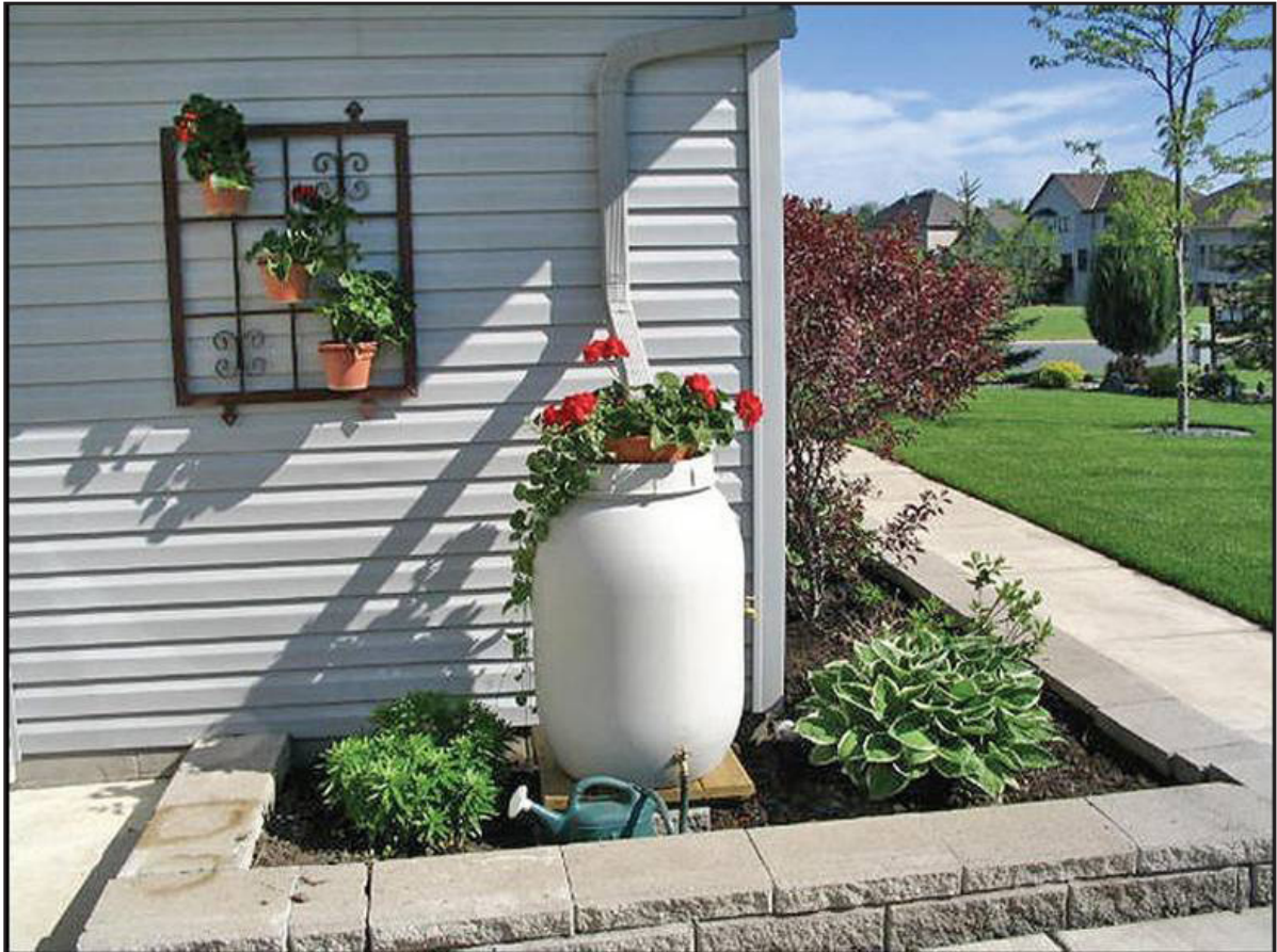
Figure 6.108: Residential Rain Barrel. Source: ABCs of MPs
