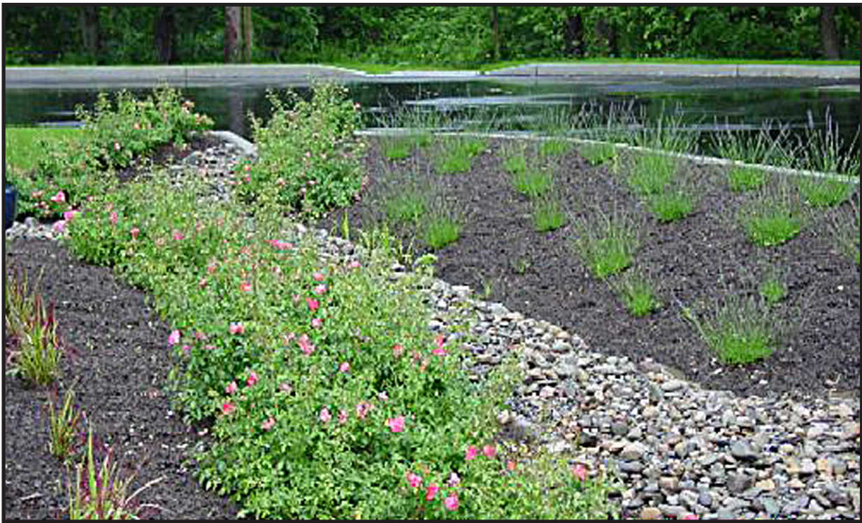
Figure 6.132: Biofiltration Infiltration Trench, Cumberland County, PA. Source: Pennsylvania Department of Environmental Protection
