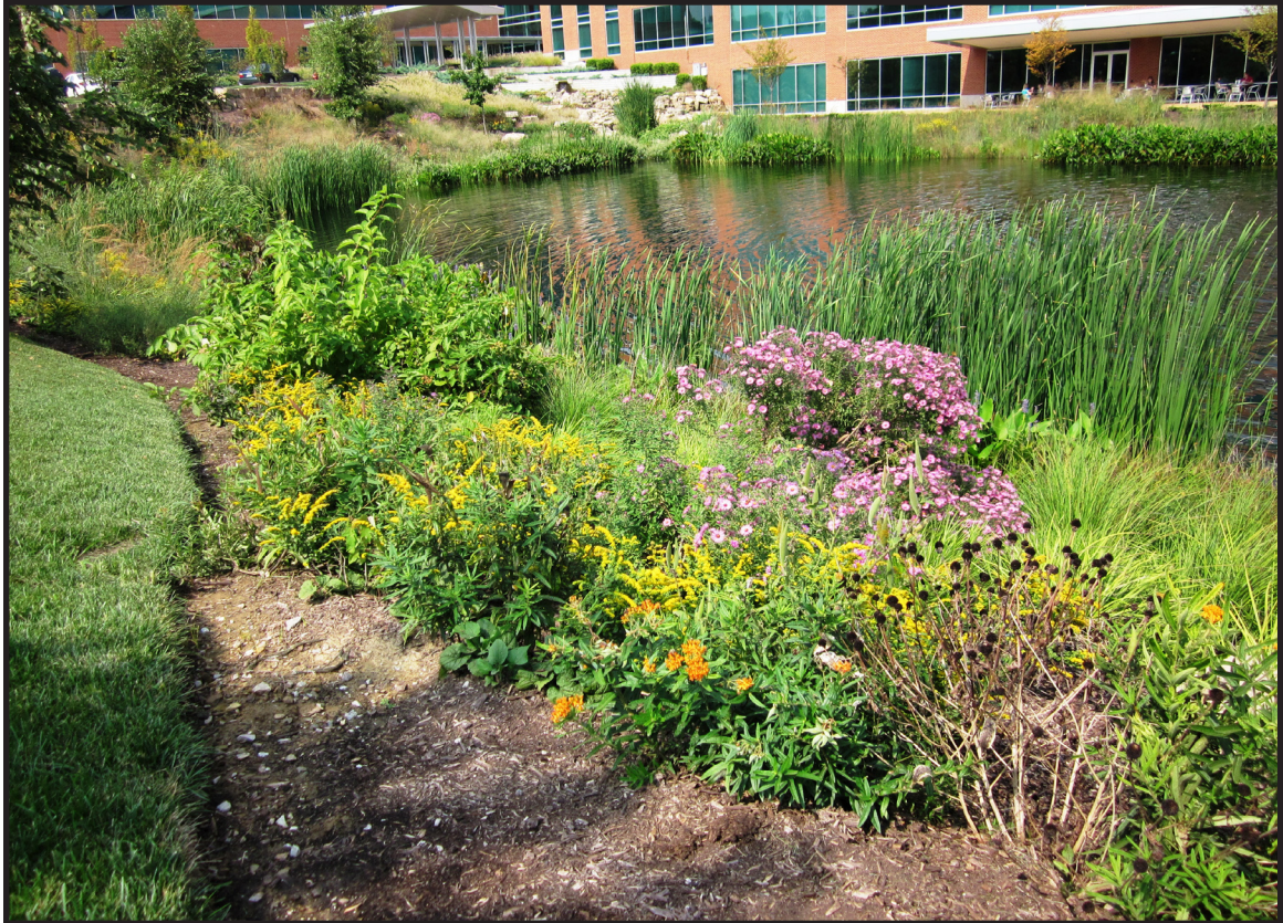
Figure 6.123: Extended Wet Detention, Express Scripts Campus, Berkeley, MO. Source: Metropolitan St. Louis Sewer District
