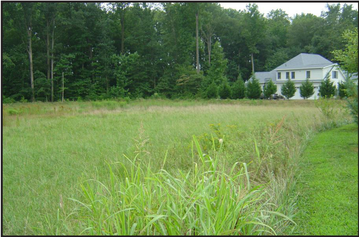
Figure 6.127: Extended Detention Wetland in a Residential Development. Dover, Delaware. Source: Kevin Magerr, PE, CPESC, CPSWQ.
