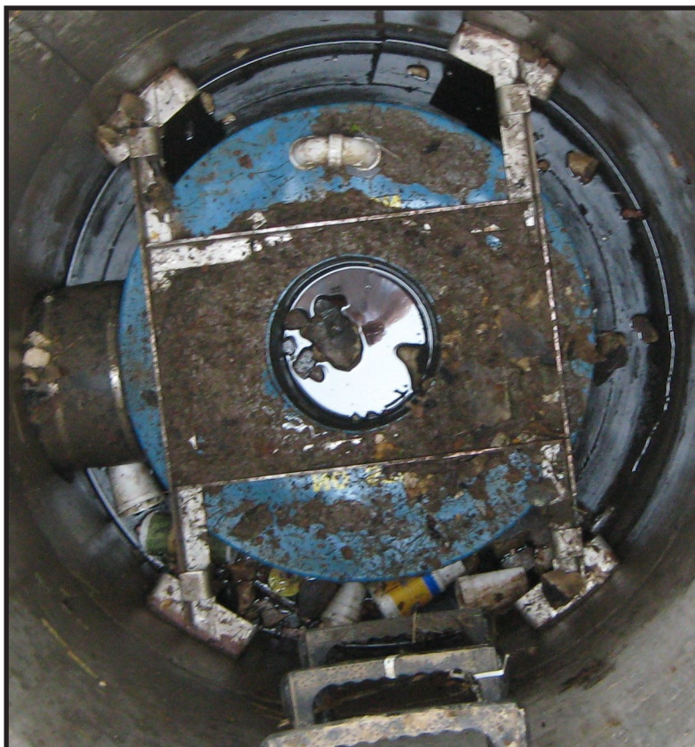
Figure 6.137: Hydrodynamic Separator. Source: MSD
