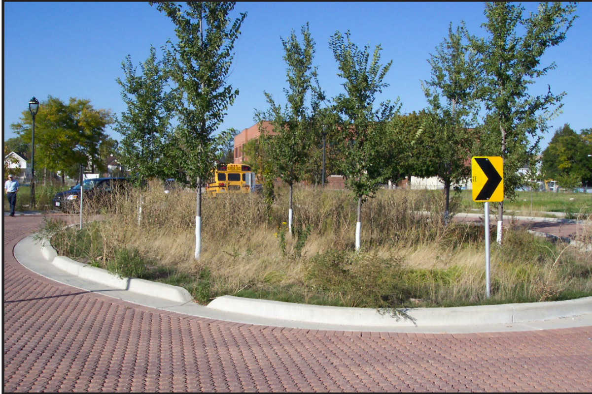
Figure 6:104 Rain garden in roundabout designed to capture/infiltrate stormwater, Milwaukee, WI. Source: Bob Newport, EPA Region 5
