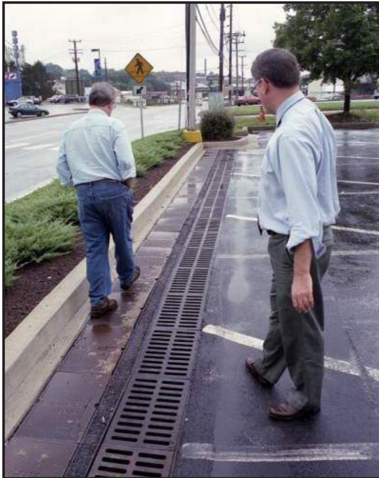
Figure 6.134: Perimeter Sand Filter. Source: Center for Watershed Protection
